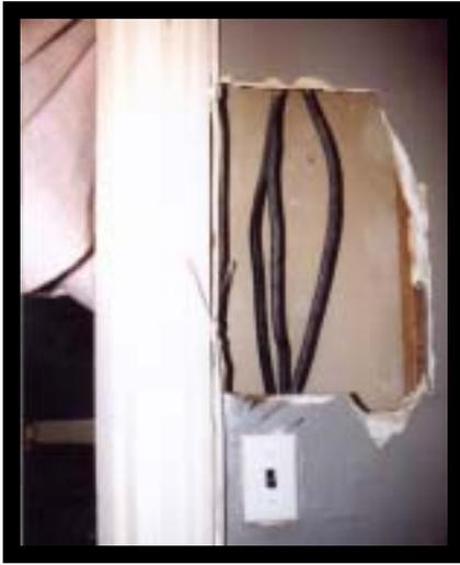
Fire separation damaged by physical abuse
