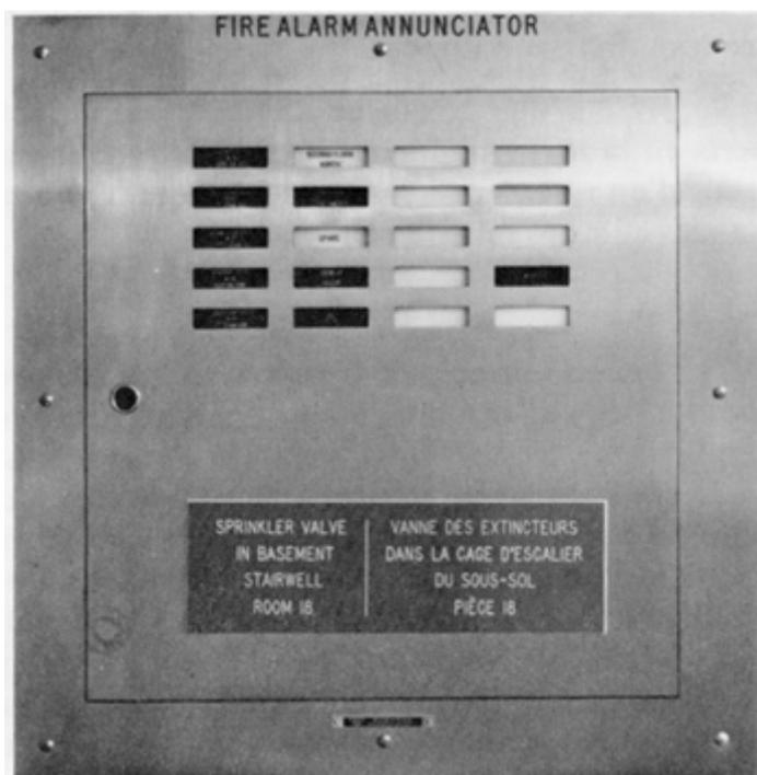
Figure 3. A typical annunciator panel with indicators for each zone of the building
